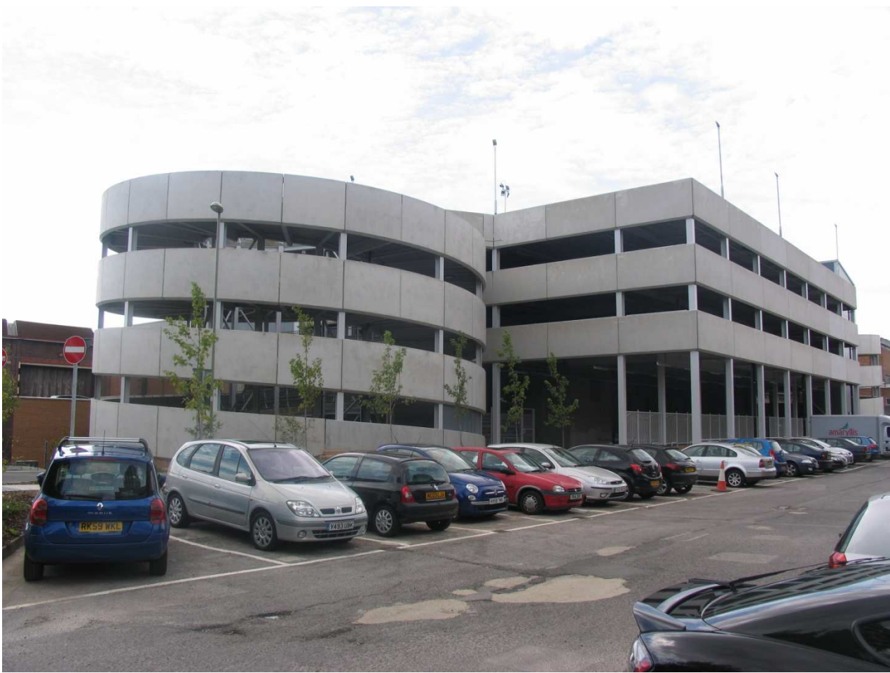
Fareham Shopping Centre Multi Storey car park
